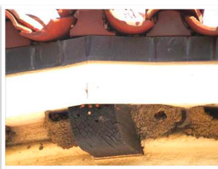
Visitor Center Eaves of Its Tower
